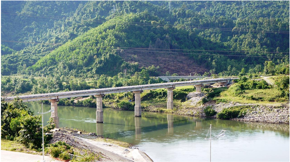
A Vuong hydropower plant in Quang Nam province of Viet Nam
